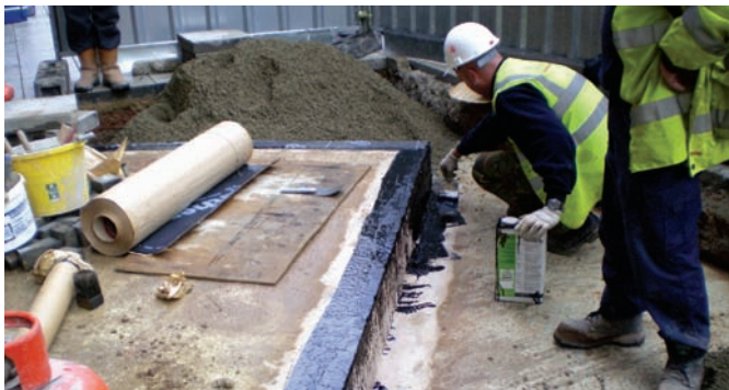
Failed waterproofing is replaced
