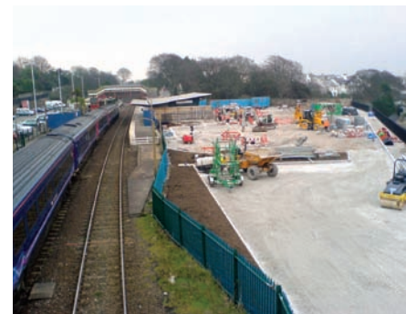
Works under way at St Austell
