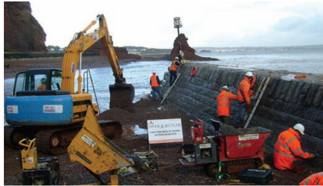
Repointing a breakwater beside the coast at Dawlish
